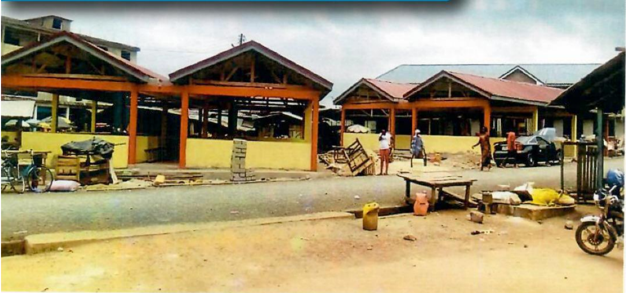
Pictures of Completed Market at Elubo in Jomoro Constituency
