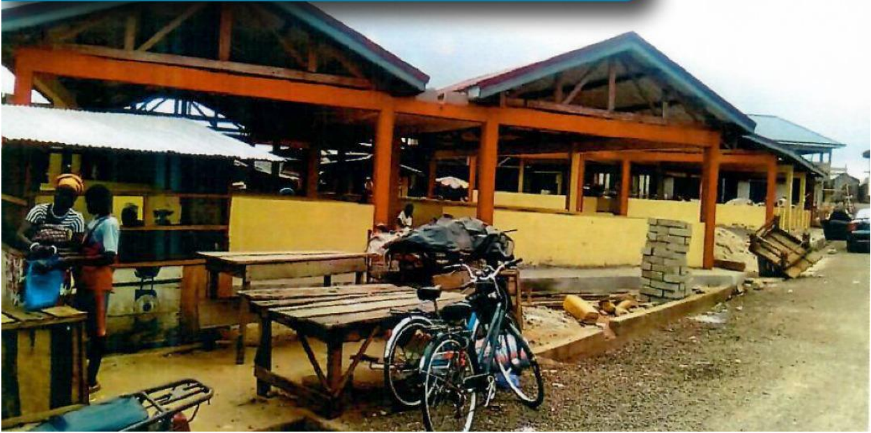
Pictures of Completed Market at Elubo in Jomoro Constituency
