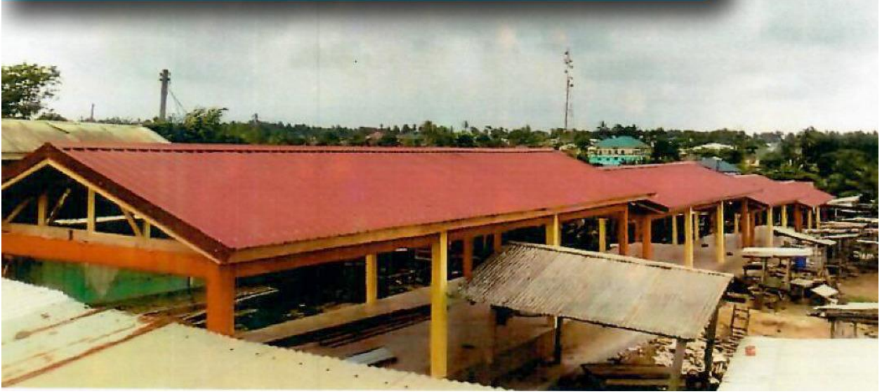
Pictures of Completed Market at Tikobo in Jomoro Constituency
